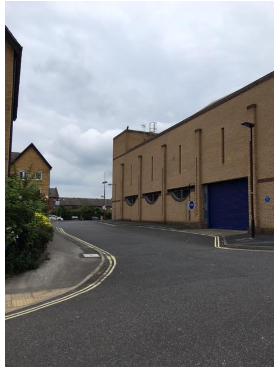
Rear Elevation Facing South/William Court
